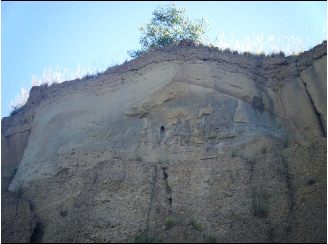
Plate 3-7: Drill Hole in South-western Rock Face of Eastern Quarry.
